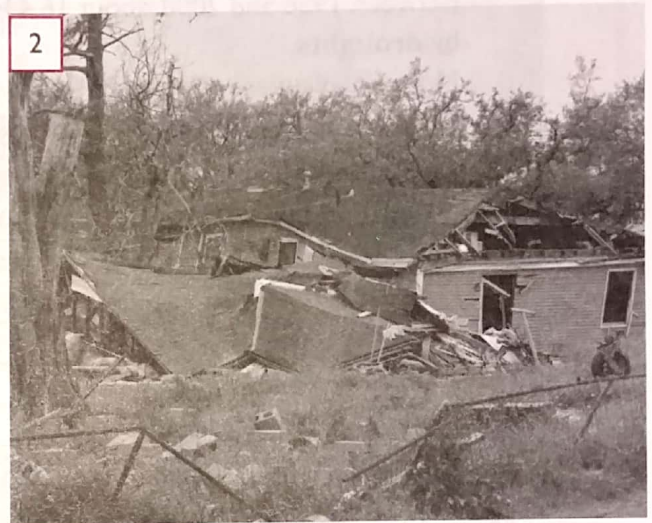
Damage caused by a hurricane
